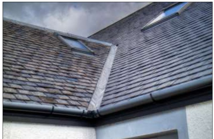
New and reclaimed slates on Community Centre
