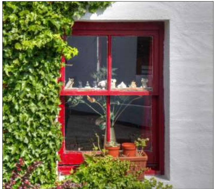
Traditional sash and case window with slim astragals—an asset to the conservation area
