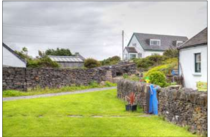
Dry-stone slate boundary walls
