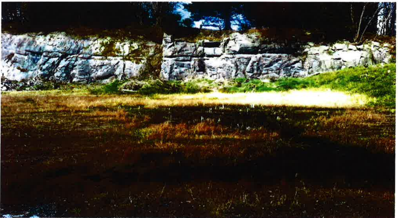
Figure 3. unstable rock face- for terracing, spoil to be moved and replaced on rocky slope once rock face is made safe. Reeds to the front to be removed and replaced once rock face treatment has been completed.
