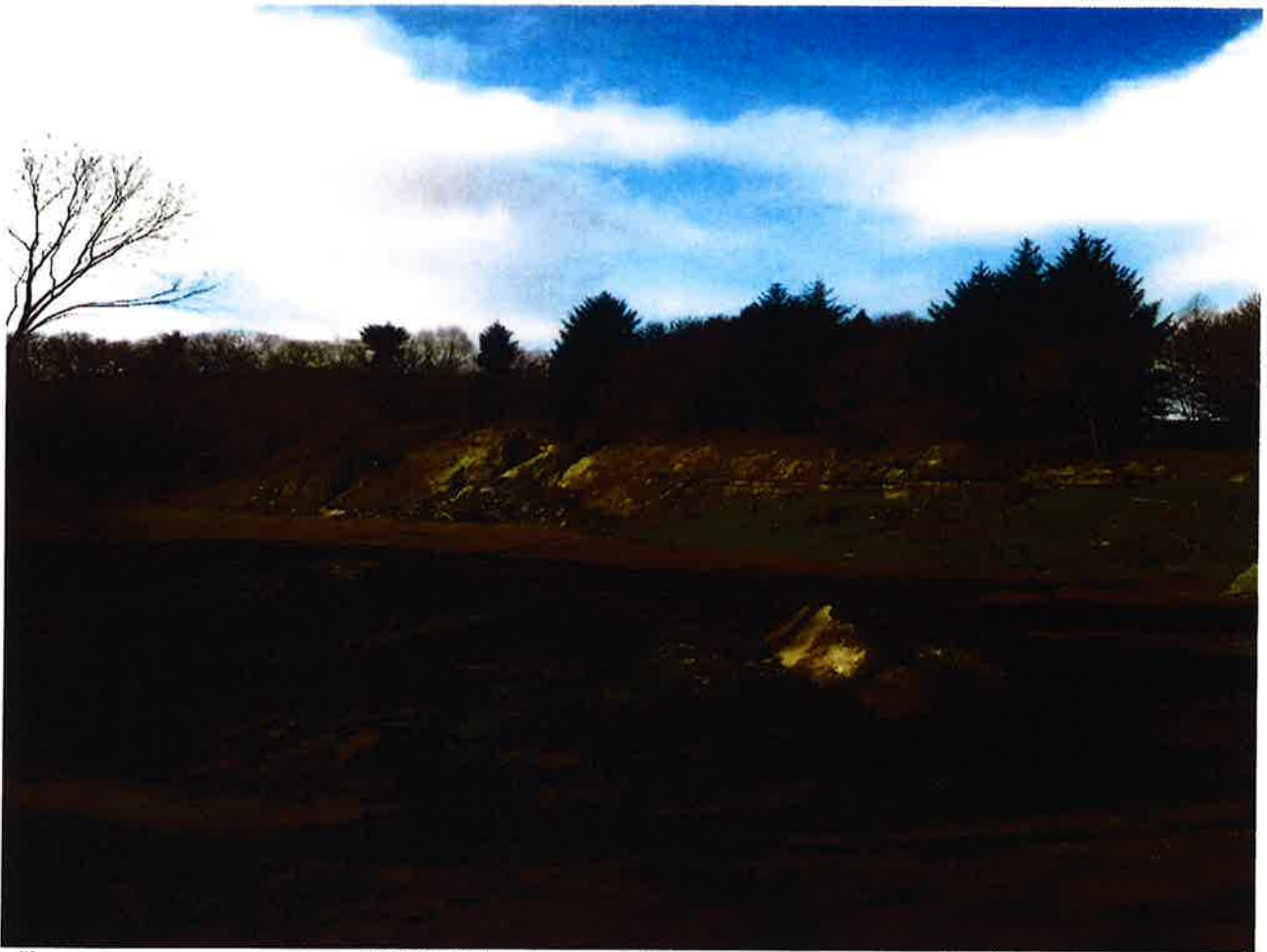
Figure 3b. View of spoil heap (right), rock pile at rock face, 30% to be moved to the front of more exposed area for terracing- see Figure 3 . Reform slope and spread soil from spoil heap. Additional rock can be taken from the existing extracted rock near the entrance or from where the excavator has been working see
