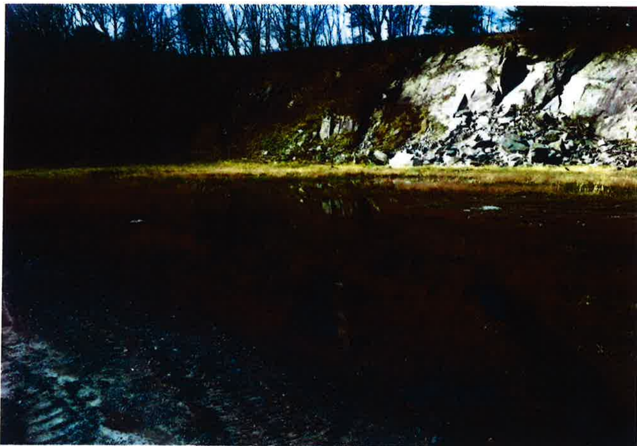
Figure 4. South west corner, Inspect rock face for loose rocks- remove and grade on slope to be made safe. Planting in corner as per Key E.
