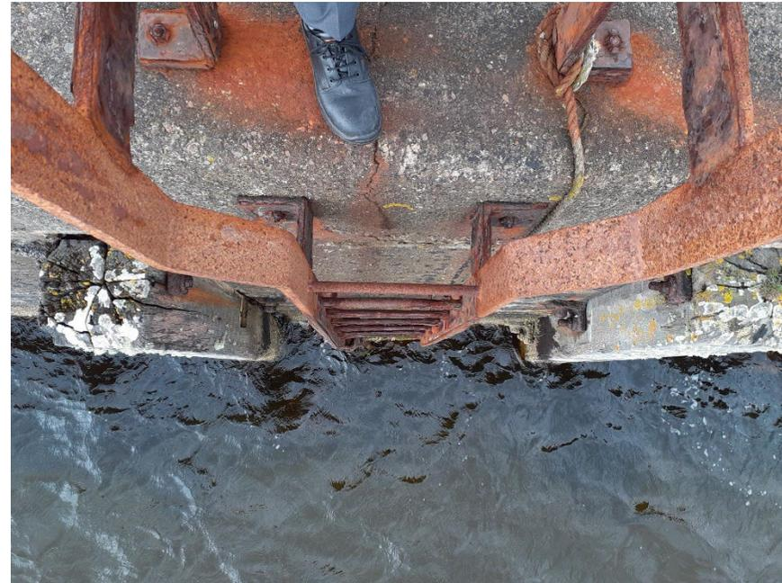
**Image B10.** Bruichladdich, severely corroded water egress ladder
