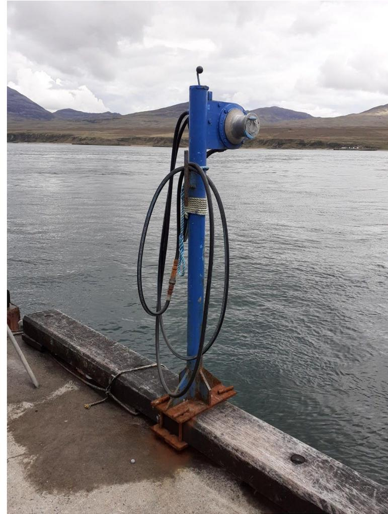
Image B8. Port Askaig, equipment inappropriately fixed
