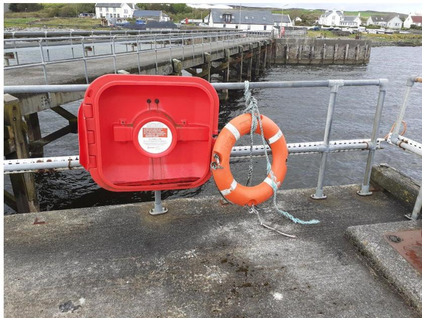
Image B11. Bruichladdich, life ring incorrectly secured
