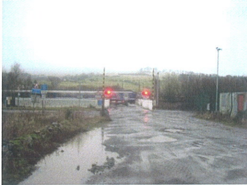
View of the level crossing on Moss Road showing working lights and barrier
