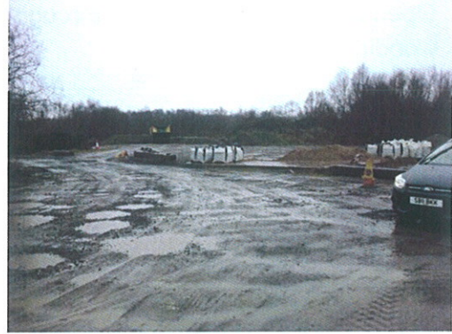
Engineering yard area
