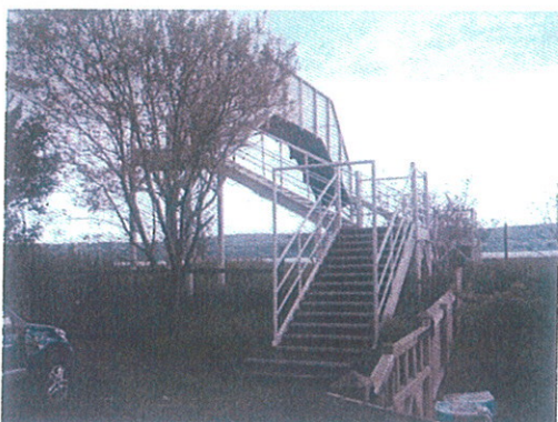
Footbridge over the Railway line at the south west end of Ferry Road.
