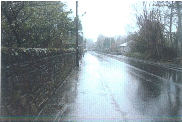
Typical wide pavement east side of the road
