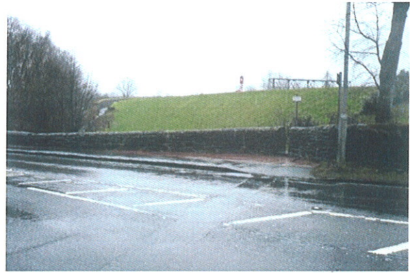
The cycle route continues on the opposite side of the road because the pavement on the east side of the road is not wide enough
