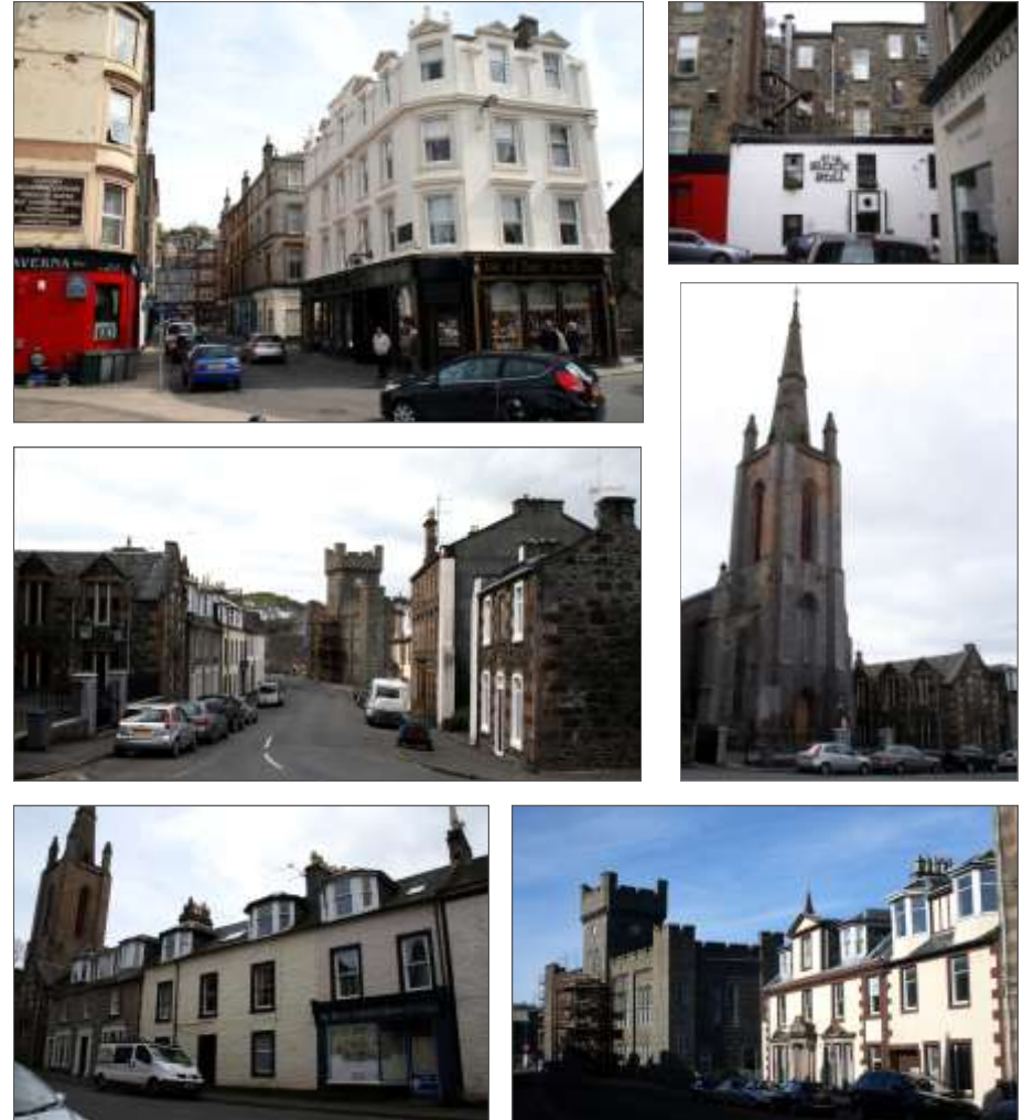
Figure 24: Top : (left) West Princes St view east from Guildford Square, note the prominent hotel buildings (left) Guildford Court Hotel and (right) Bute House Hotel; (right) Black Bull on West Princes Street; Centre: (left) Castle Street looking west from the junction with Bishop Street which is marked by the spire of Trinity Parish Church (right); Below: (left) 2-storey buildings on Castle St; (right) listed houses at Nos 7-9 with refinement, beyond the former County Buildings mark the corner with High Street.
