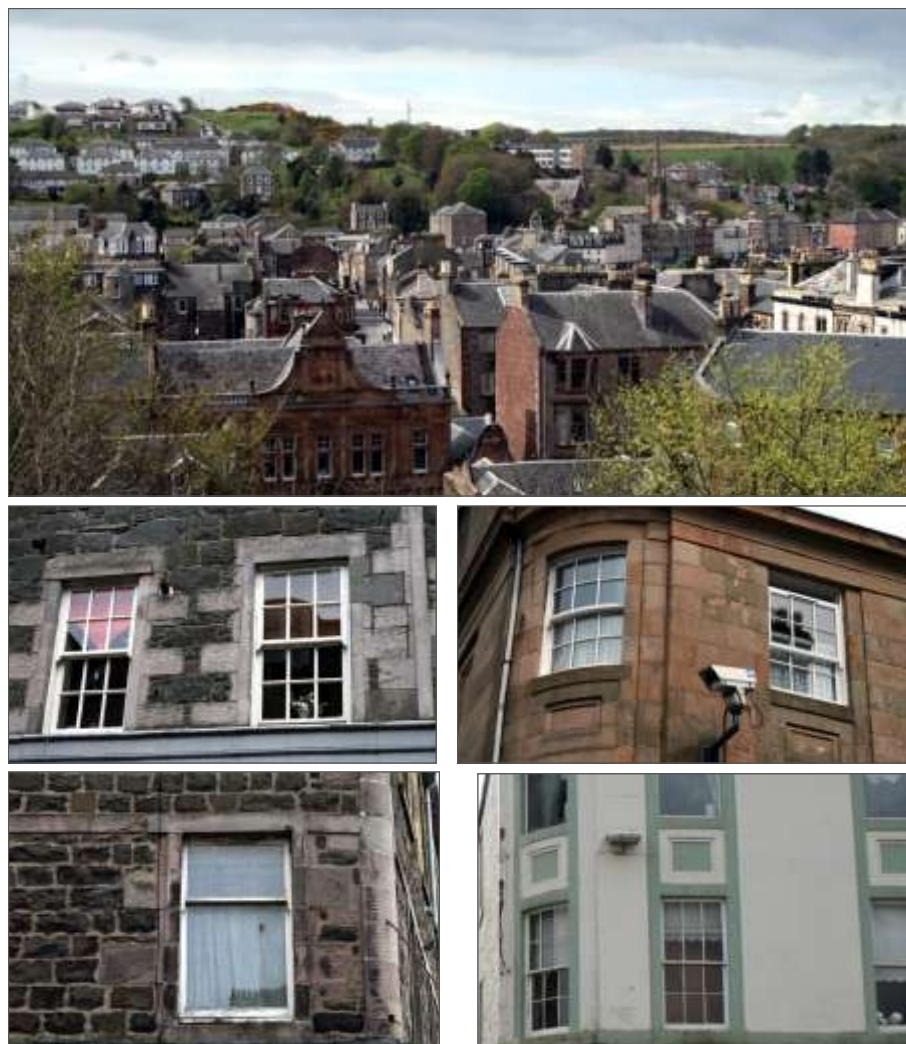
Figure 34: Top: a view over the town illustrates the predominance of traditional pitched and slated roofs; the variety of stone colour intermingles with lightly coloured painted facades; Centre & Below: (left) stonework with contrasting use of sandstones & whinstone with dressed window surrounds and corner quoins, these may have originally been lime rendered; (right) others have finer dressed sandstone which with no margins was not designed for render. Some of these buildings have now been painted.
