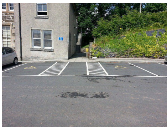
Accessible entrance right hand rear of building
