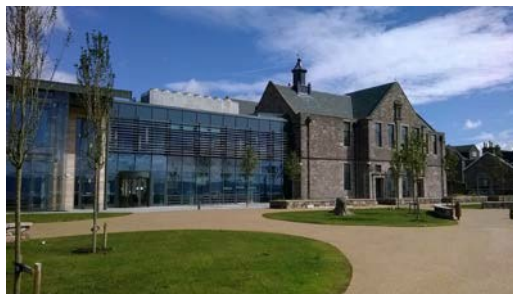
Accessible entrance at front of building
