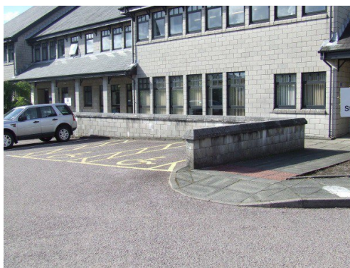
Accessible parking bays and ramp leading towards the main entrance on the left
